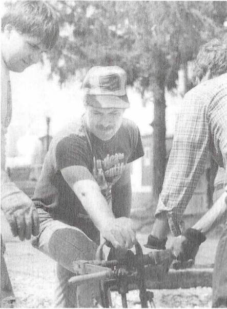
Greg Vertein, John Sorrel, and Jay Slide work on the Walnut St. crossing during the Spring Fling weekend.
