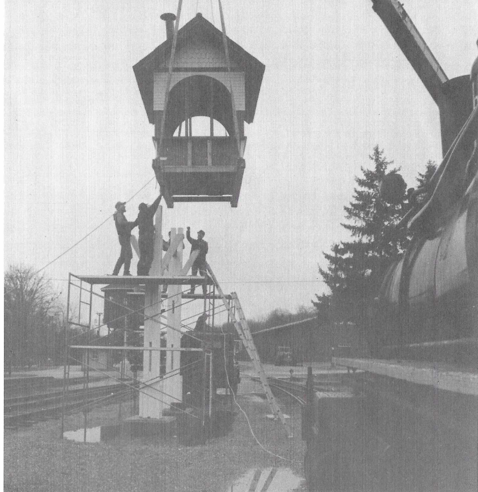
Mid-Century volunteers carefully guide the tower into position. Dan Griffith (page 8) and others firmly fasten the tower to the frame.
