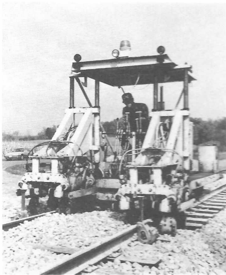
Jeff Nelson, superintendent of the engineering department, works on Mid-Continent's tamper at Ulrich Road.
