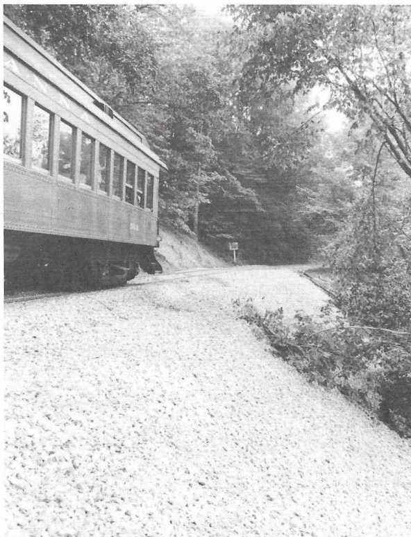
A trackside view shows the extensive repairs to stabilize the bank after the big rain.
