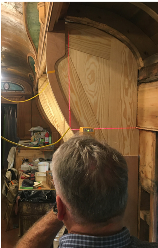
Test fitting the berth partition trim piece in the sleeping compartment with the aid of a laser
