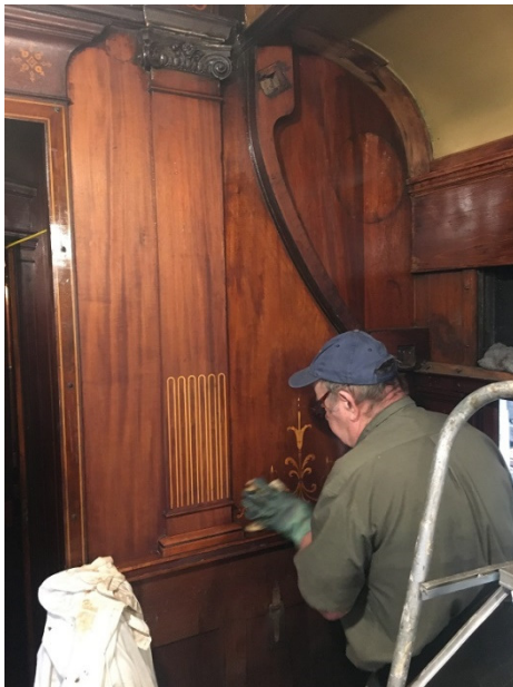
Interior woodwork in the process of being stripped inside the DULUTH
