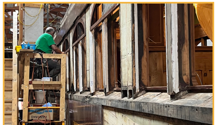
The letter board and arched windows in the process of being filled (epoxy) and sanded.
